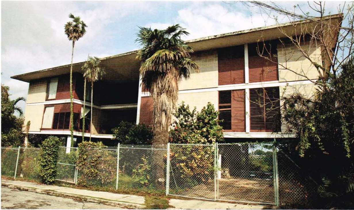
Top: The house is raised on pilotis above the ground floor, defining a covered terrace, space for parking, a service area, and the entry stair. The shaded vertical recess separates the public and private zones of both upper floors.
